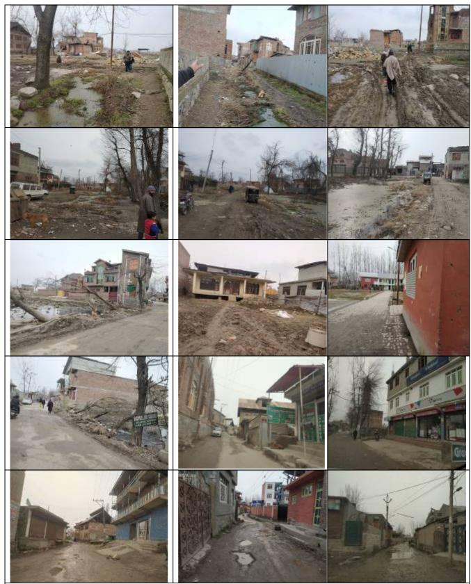
From Palpora-Noorbagh to Palpora-Goripora, the existing road condition and persistent water logging results into degradation of road surface due to the non-existence of the efficient drainage system. People are suffering on daily basis which has resulted into the negative social and environmental impact in the whole area.
